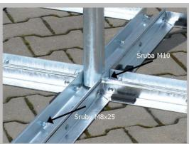
3. We fasten the flat bars to reinforce the structure.
